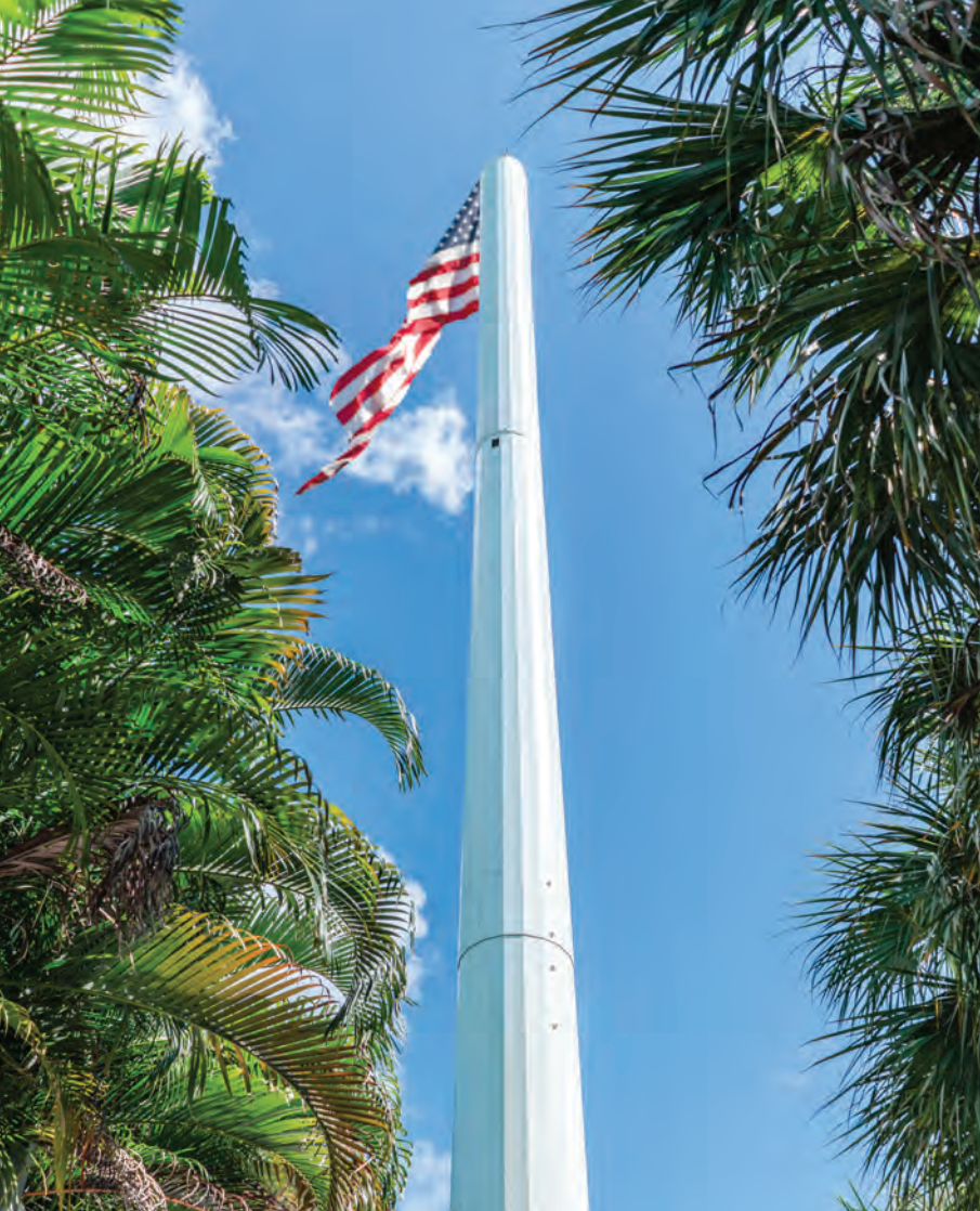
▼ Hiding in Plain Sight (clockwise from bottom left): Vertical Bridge's stealth structures include a "monopine" tower in Alaska; a flagpole tower in Florida; a "monopalm" tower in Texas; and a "guyed" tower in Colorado
